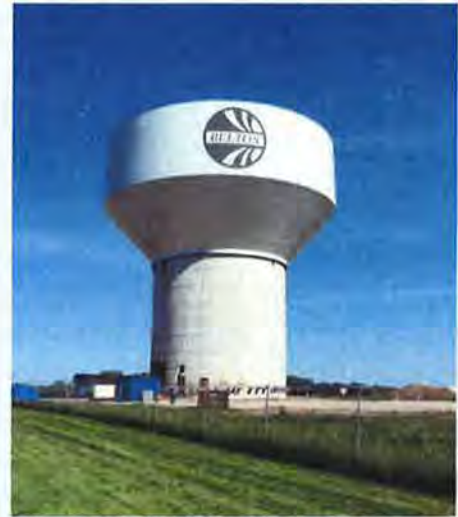
Figure 1. New 3 million gallon Water Tower
