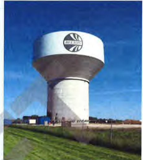
Figure 1. New 3 million gallon Water Tower
