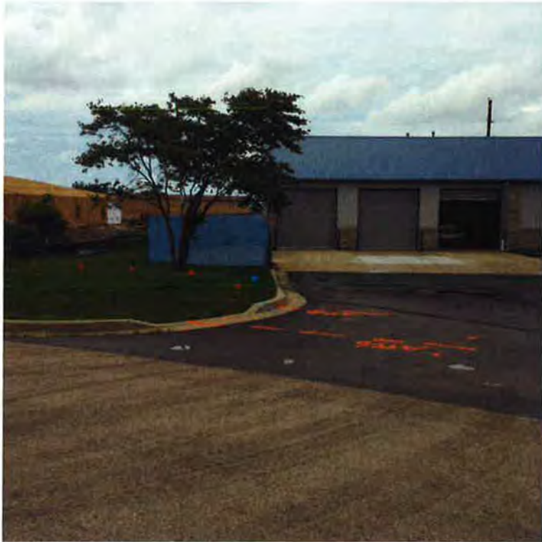
Photo 1. Facing north toward Rudroff Building – no utilities along existing easement to be vacated
