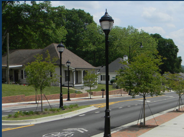
SPECIALTY STREET LIGHTING
