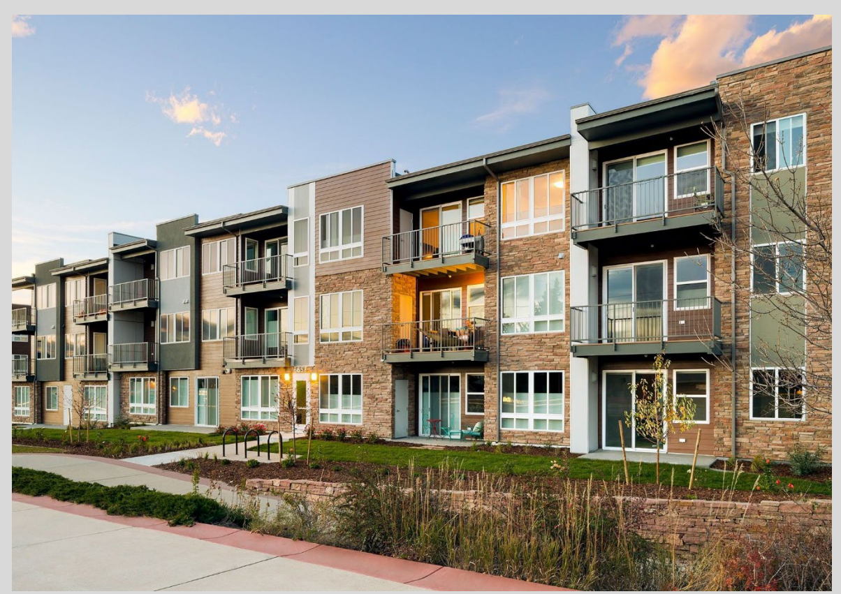
THREE-STORY MULTIFAMILY HOUSING
