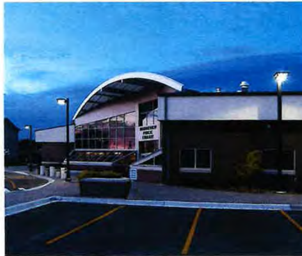
FIGURE 1.06 EXTERIOR LIGHTING EXAMPLES
