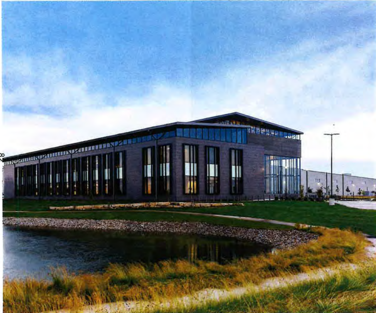
FIGURE 1.07 QUIK TRIP DISTRIBUTION CENTER, BELTON, MISSOURI
