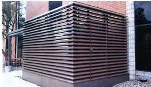
FIGURE 1.14 EQUIPMENT AND TRASH SCREENING EXAMPLES
