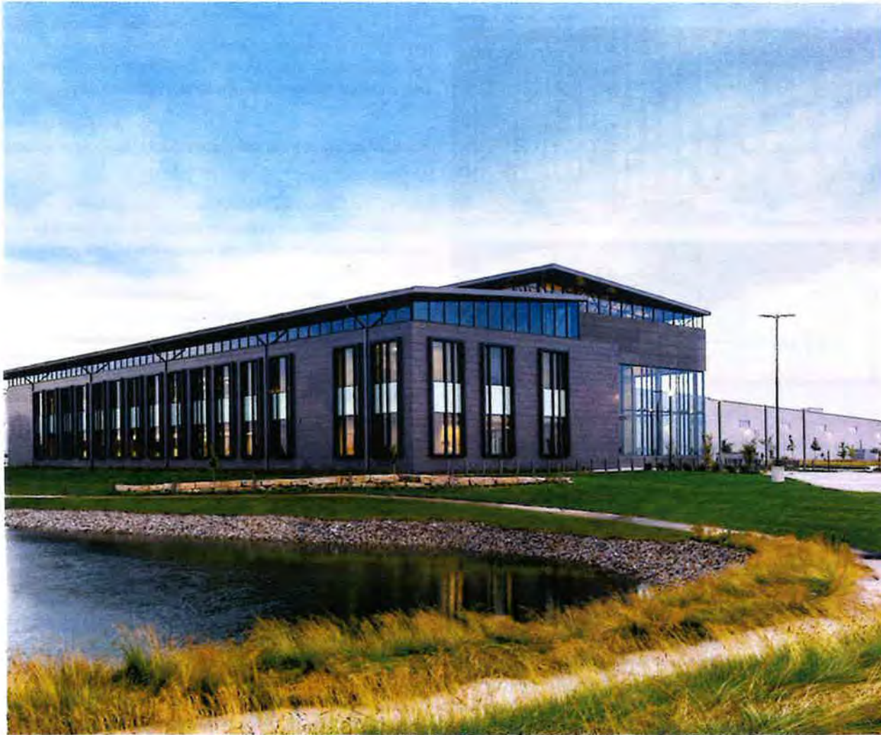
FIGURE 1.09 QUIK TRIP DISTRIBUTION CENTER, BELTON, MISSOURI
