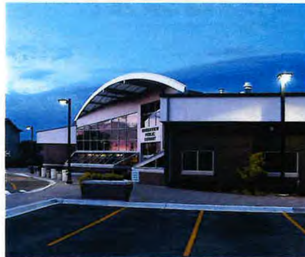
FIGURE 1.08 EXTERIOR LIGHTING EXAMPLES
